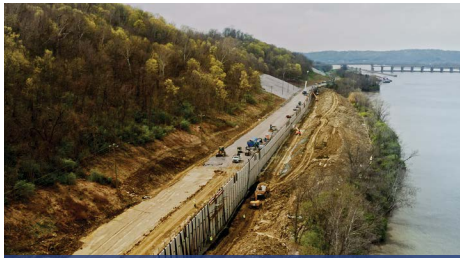
GALLATIN COUNTY SLIDE REPAIR | WARSAW, KY
