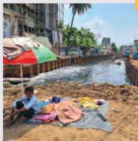
Construction of box drains with road in Cuttack city of Orissa state in 2021 & 2022.
