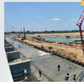
Rehabilitation of Kattalai Barrage near mayanur in Karur District of Tamil Nadu in 2022.
