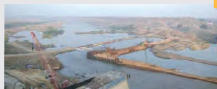
Cofferdam for Varkhede-Londhe barrage foundation on Girna River at Chalisgaon in Maharashtra in 2018.
