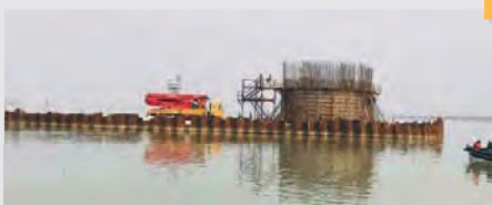
Cofferdam for well sinking for new six-lane bridge over Ganga river near Kachchi Dargah in Patna, Bihar in 2018.
